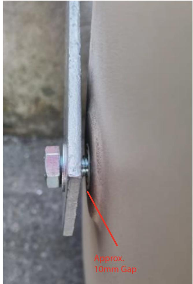
Please follow the installation drawing for the Wall restraint kit, use all 4 wall brackets for each tank
